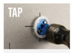
Use a hammer to gently tap the fixing into the drilled hole.
