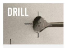
Use a flat drill bit to drill a hole in the plasterboard.
